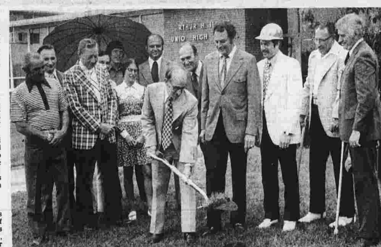
Dual Ground-Breaking for School Additions Twin ground-breaking ceremonies were held in the rain Friday for renovations and additions to Iling and Bennett Junior High Schools, under a $5.6-million appropriation approved last November in referendum.
